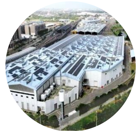
Taoyuan MRT Qingpu Solar Photovoltaic Plant
