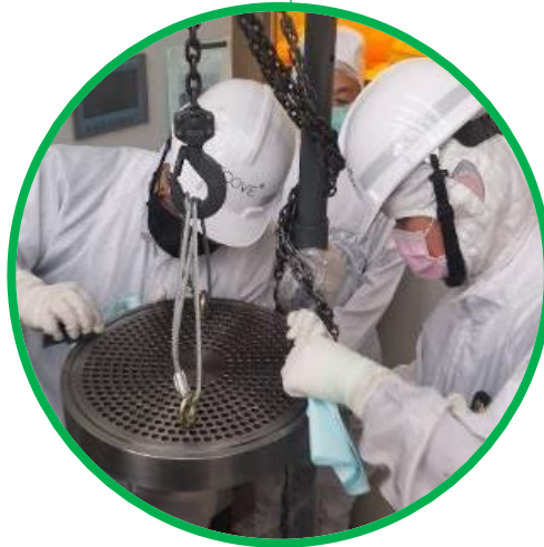
Cleanroom process equipment maintenance
