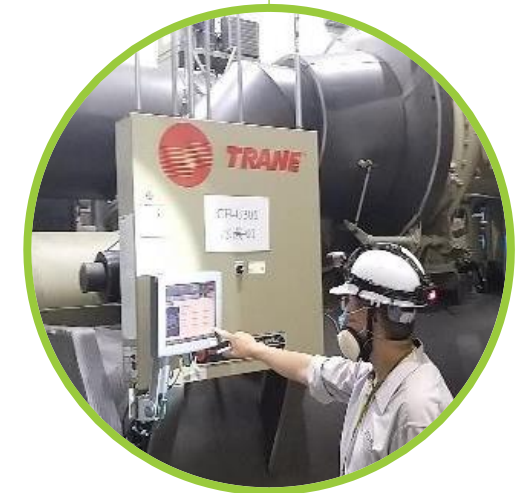
Chiller equipment maintenance
